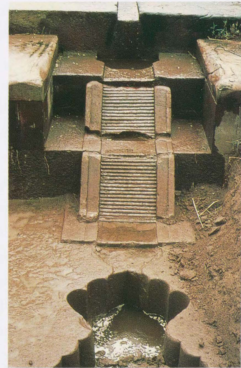
Water chute between two rock-cut lotus pools on the main terrace, Lotus Garden at Dholpur, 1978. Photograph by Elizabeth B. Moynihan
