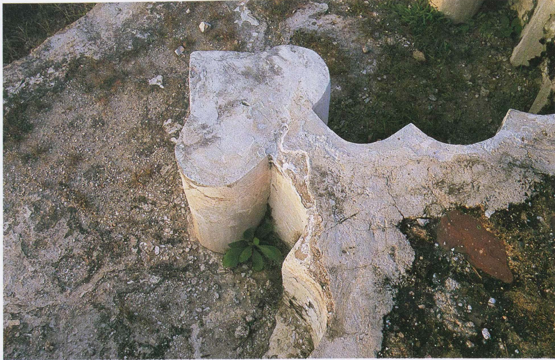
Figure 8. Dilapidated sandstone lobe from the octagonal pool on the riverside terrace, 1999. Photograph by Neil Greentree
